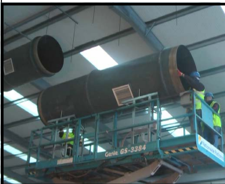
Ductwork being installed at the Rochdale site
