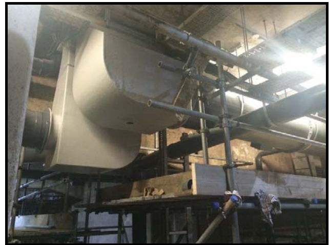
Fig 7 - Underground ductwork – accessed from scaffolding above the live inlet channel
