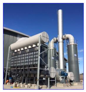
concentration at the stack – designed to maximise carbon bed life and minimise pressure drop (and therefore the power consumption by the fan).
