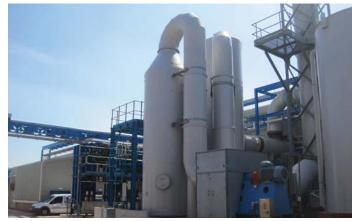
The materials of construction for the treatment plant had to be considered very carefully due to the highly corrosive (HCl) nature and temperature of the gas stream. The ceramic filter, the sub cooler and the RTO were constructed in Hastelloy C22, a high grade steel.
