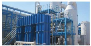
The high temperature of the gas meant that only a ceramic filter would be able to remove the majority of the entrained fibre content - protecting the downstream equipment from clogging.
