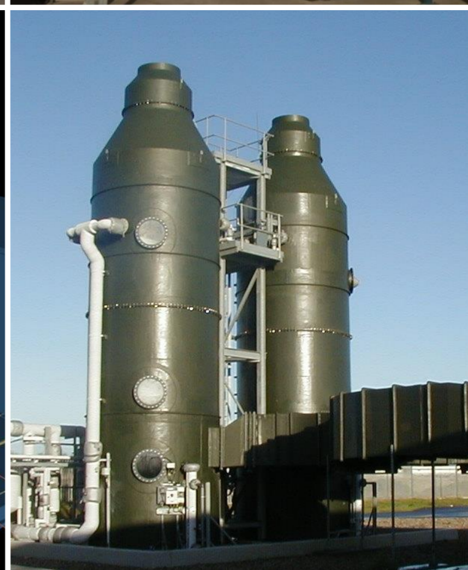
Plant model showing scrubber
