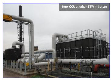
The new main OCU comprises a bio-trickling filter and carbon filter polish to achieve the odour discharge of 1,000 ou<sub>E</sub>/m³ with all equipment drawn from ERG's standardised range to Southern Water and WIMES standards. ERG completed this project in early 2020.
