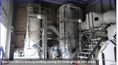
odorous air from the Works was possible while ERG installed the new ductwork, scrubbing package, fans and chemical storage. Here again, ERG designed and installed significant temporary ventilation and odour control to permit safe working and secure odour treatment during the installation phase.
