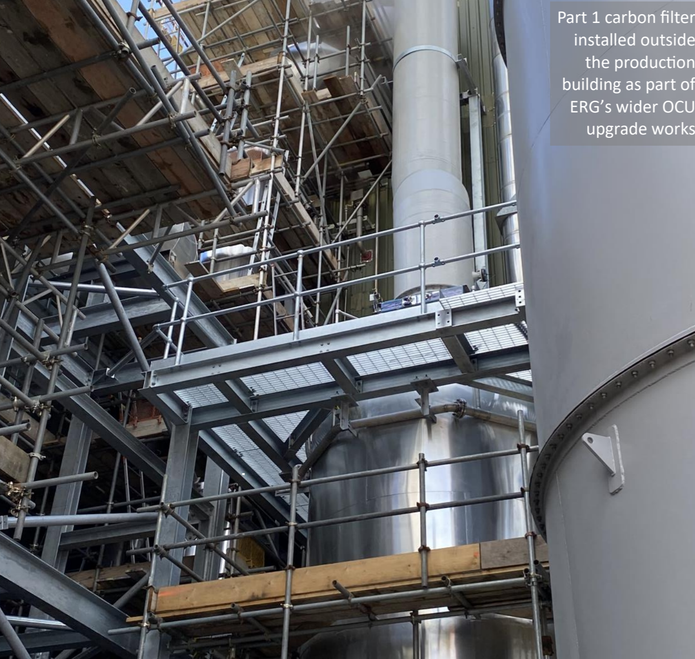
Original 1990s scrubber upper section rotated to accommodate ductwork to the heater and carbon filter, then ducted back to the original stack
