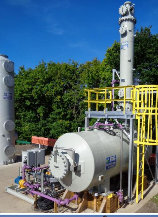
Complete package installed on site including the quench, wet scrubber, carbon filters, fan, stack and access structure
