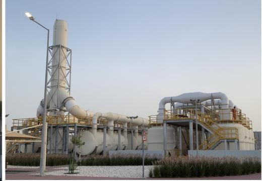
Bio-trickling filter and associated isolation dampers, recirculation liquor pumps and pipework with steelwork mounted at -4m level
