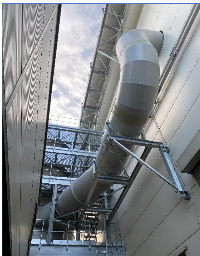
System 2 ductwork installed at 8m above grade
