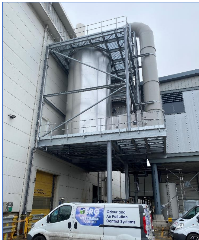
System 2 installed on a platform at 5.5m level. Reheater and carbon filter visible with scrubber vessel behind
