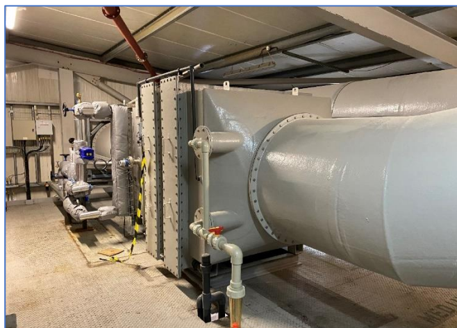
System 3 demister and steam-fed heater prior to carbon filter
