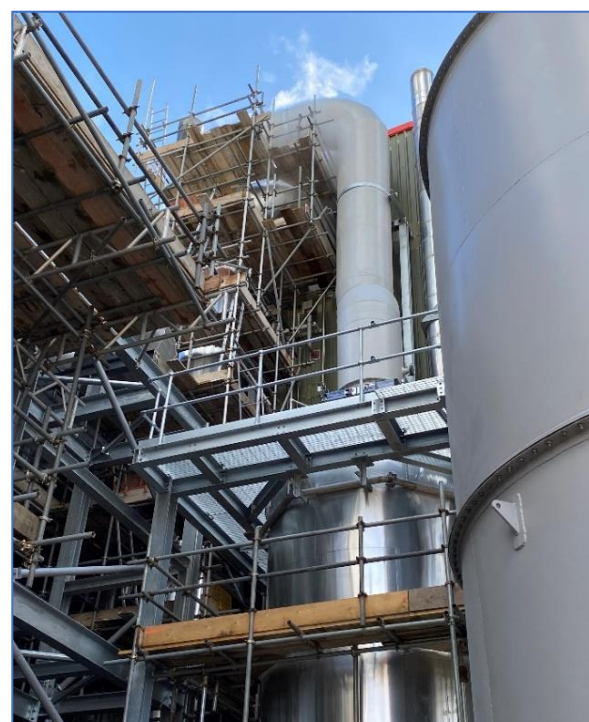
System 3 carbon filter installed during phase 1
