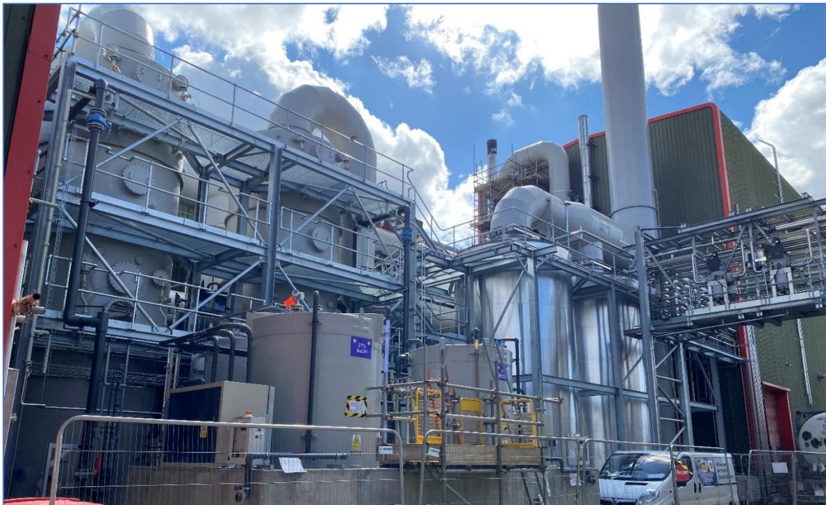
One of three new odour control systems on the site ("system 1"): two parallel streams, chemical scrubbers followed by carbon filtration. Package includes access steelwork, chemical storage/dosing, ductwork, stack, MCC and controls
