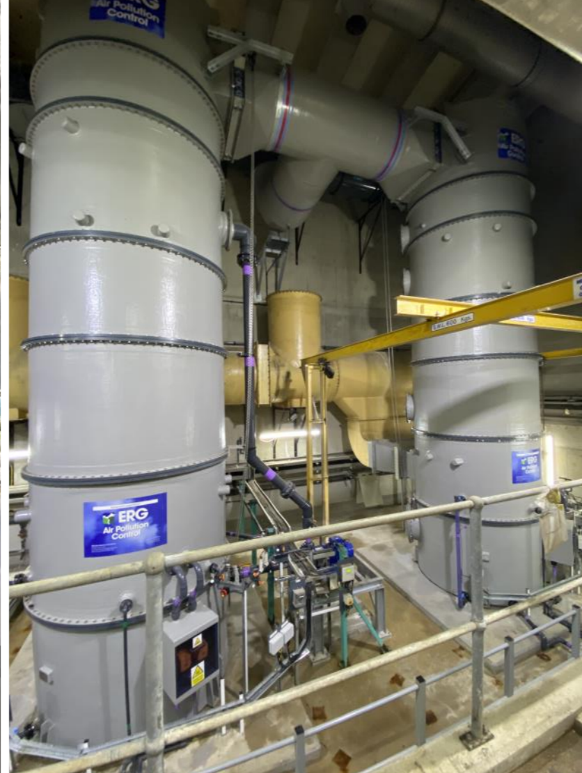
The two new scrubbers are smaller than the original vessels and achieve the same treatment standard of <250ppb H 2 S.
