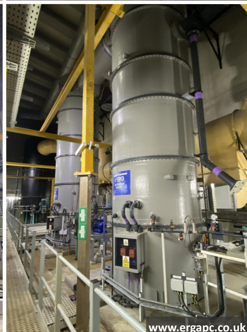
ERG's new scrubbers were manufactured in sections to suit the doorway into the OCU room in this underground sewage works and were designed to tie-in with the original ductwork connections.
