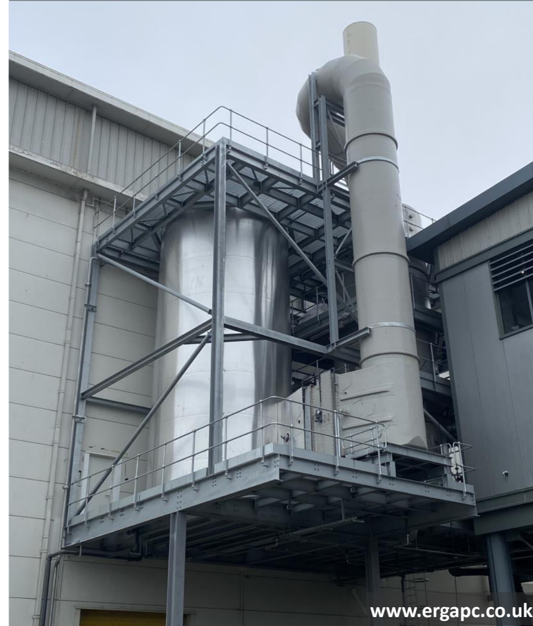
2-stage chemical scrubber, heater and carbon filter on raised platform above existing access route on site. Access and support steelwork supply and installation in ERG scope. Scrubber recirculation pumps and 2nd stage recirc tank installed at grade. Control panel and chemical storage & dosing equipment installed inside the building.
