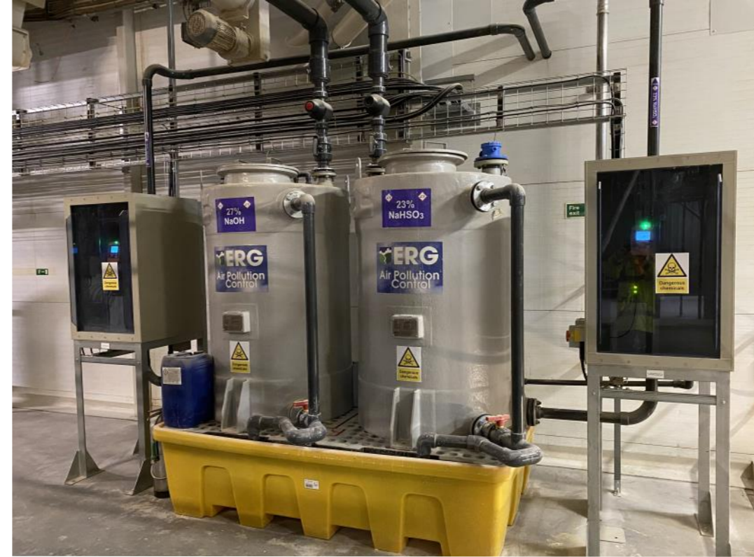
2-stage chemical scrubber, heater and carbon filter on raised platform above existing access route on site. Access and support steelwork supply and installation in ERG scope. Scrubber recirculation pumps and 2nd stage recirc tank installed at grade. Control panel and chemical storage & dosing equipment installed inside the building.
