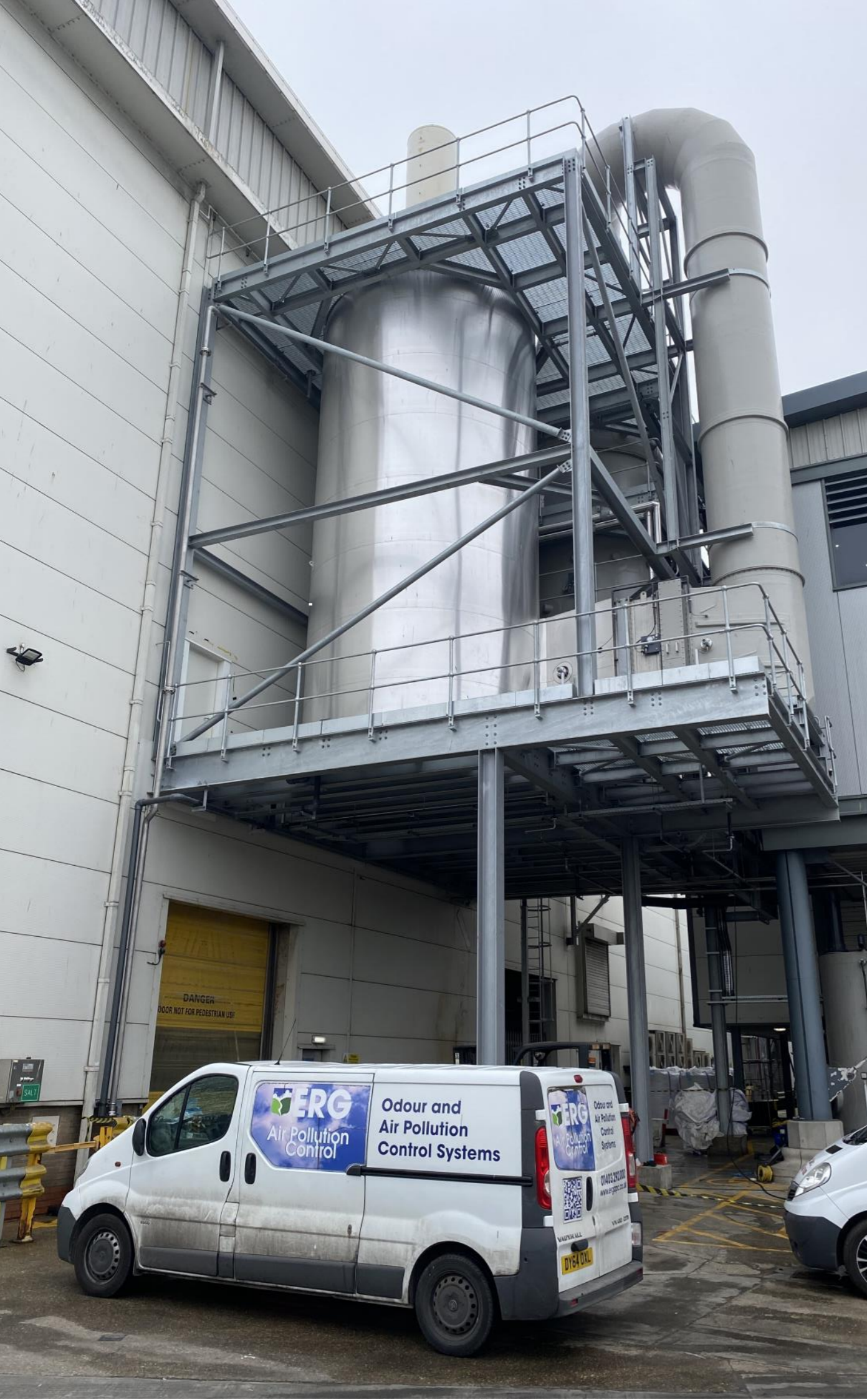
2-stage chemical scrubber, heater and carbon filter on raised platform above existing access route on site. Access and support steelwork supply and installation in ERG scope. Scrubber recirculation pumps and 2nd stage recirc tank installed at grade. Control panel and chemical storage & dosing equipment installed inside the building.
