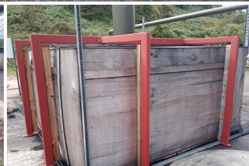
Temporary filter reduces plant downtime after existing equipment was fire damaged
